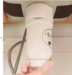
*\*Important note: Hand tighten, ONLY. Do not use wrench on plastic housing or nut.*
